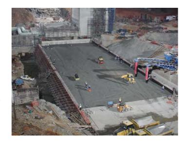
The dam foundation was investigated during the design phase using specialised geophysical techniques and core drilling. The design founding level and the final founding level after excavated during construction were similar due to the proper investigations.
